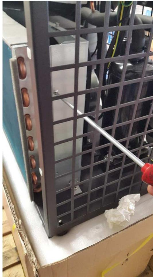
*Remove the 2 screws mounted alongside the condenser, using the screw-driver (as shown in the picture).*
